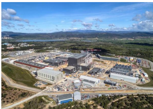
Figure 12. ITER Site – Construction in progress (Source: ITER Organization)
