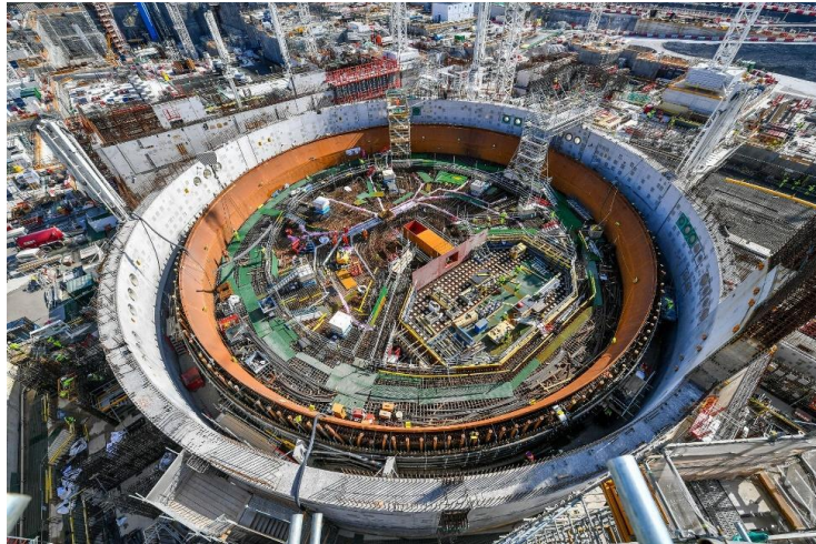
Figure 11. AP1000 in Construction – Containment Bottom
